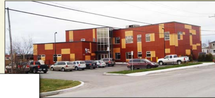
Day Care Facility
