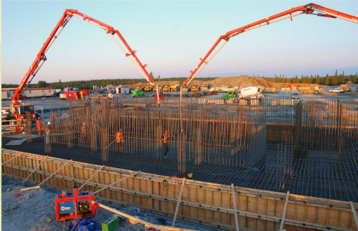
Sag Mill Foundation Preparation
